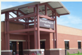
Drumright Hospital 610 West Truck Bypass Drumright, OK 74030 Daryl Morris 918.382.2300
