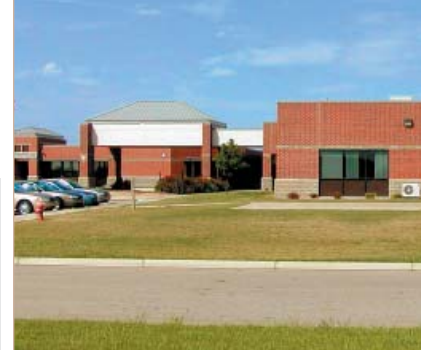
Ellsworth County Medical Center Ellsworth, Kansas
