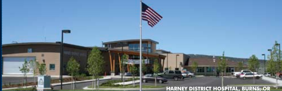
HARNEY DISTRICT HOSPITAL, BURNS, OR
