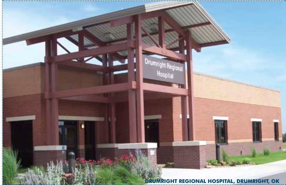
DRUMRIGHT REGIONAL HOSPITAL, DRUMRIGHT, OK
