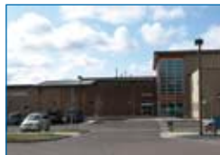
Harney District Hospital 557 West Washington Burns, OR 97720 Jim Bishop 541.573.8329
